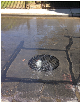
Picture of District SSO that took place on June 16, 2014, due to a blockage caused by FOG.
